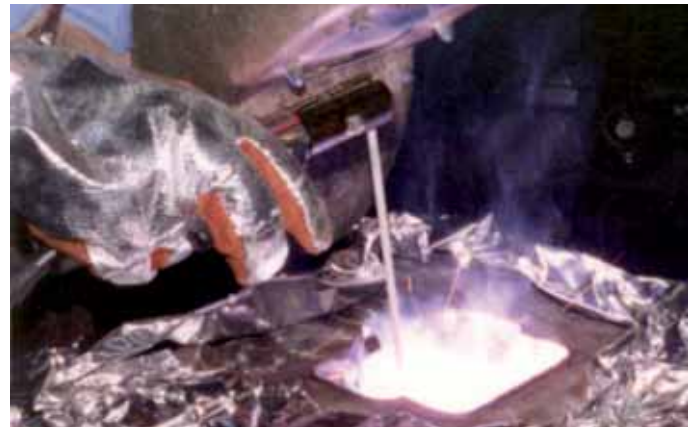
Manual arc welding and covering of components
